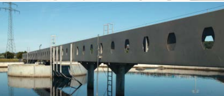
Stormwater tank (above) and sewage treatment plants (below) help to provide clean water.
